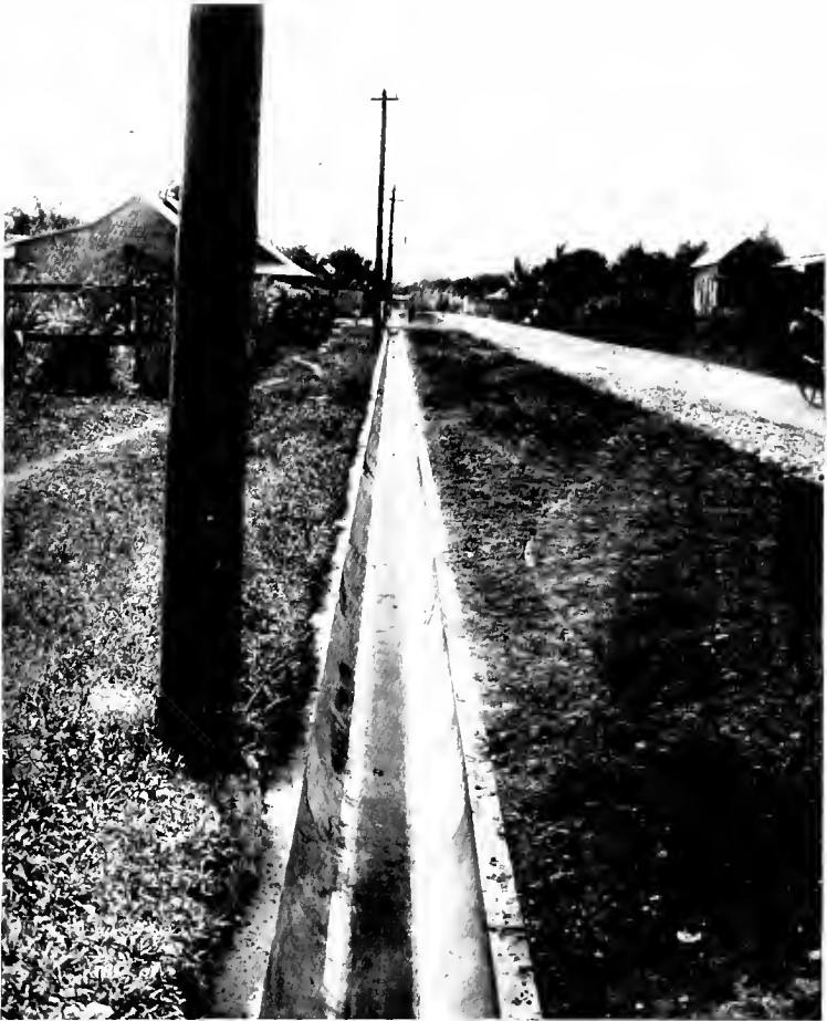
FIG. 29.—A CONCRETE ROADSIDE DRAIN, PORT OF SPAIN, TRINIDAD.
